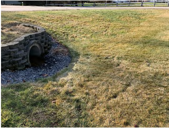
29 Gundalow - 1 (Drainage Area)
