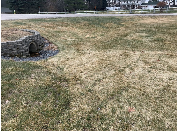
29 Gundalow - 1 (Drainage Area)
