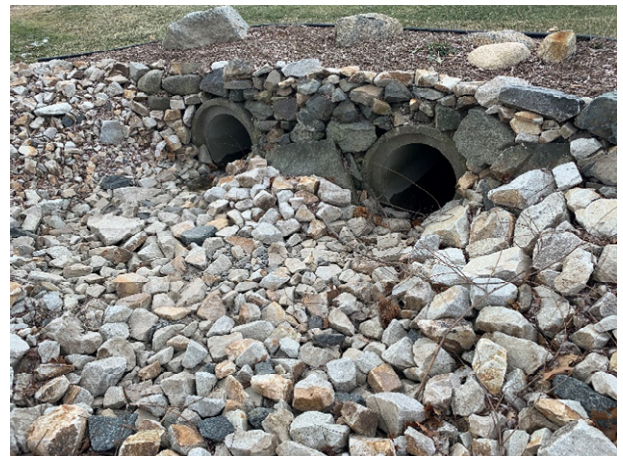
64 Gundalow - 2 (Drainage Course)
